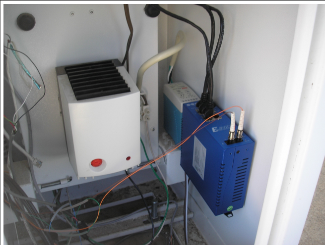
Ethernet hardware in TICO
