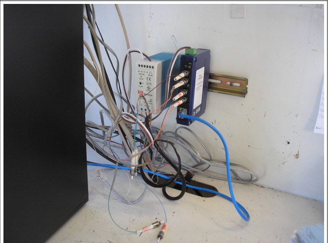
Ethernet hardware in shack
