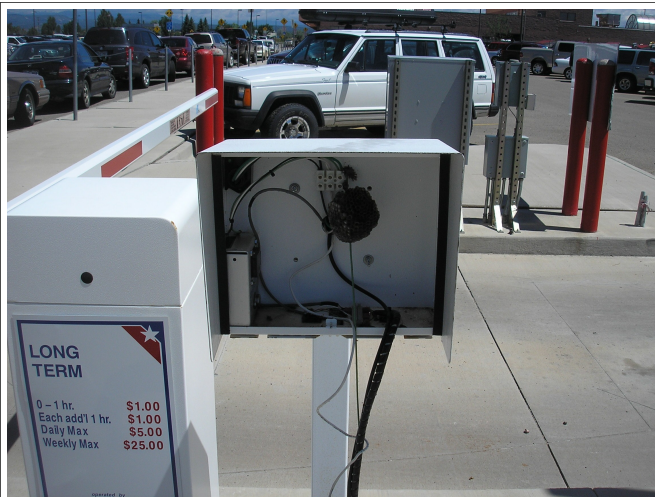
Entrance Station, showing wasp nest
